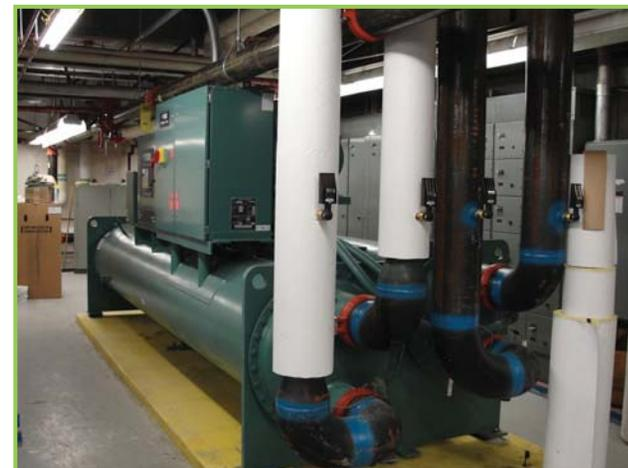
Two new energy efficient water-cooled chillers were recently installed in the the County Campus. These two chillers will save approximately \$11,500 per year in energy costs.
