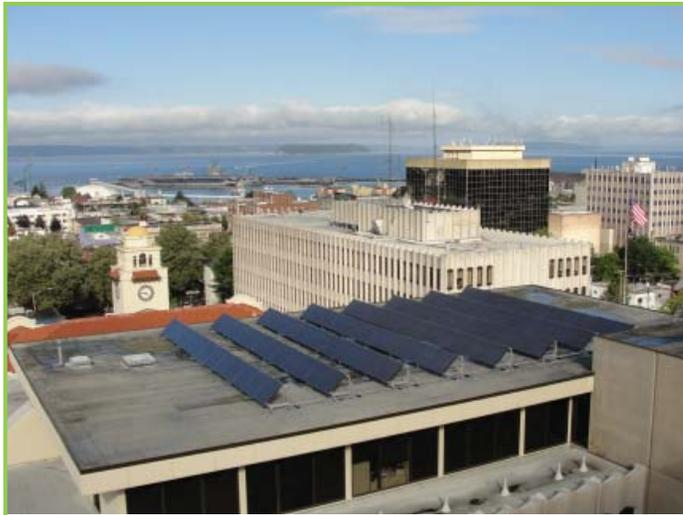
A 16.4 kW solar panel system was recently installed on the roof of the County campus administration building. This solar array will generate electricity for approximately 16 electric vehicle charging stations in the County parking garage and will prevent approximately 21,000 pounds of CO2 from entering the atmosphere each year.
