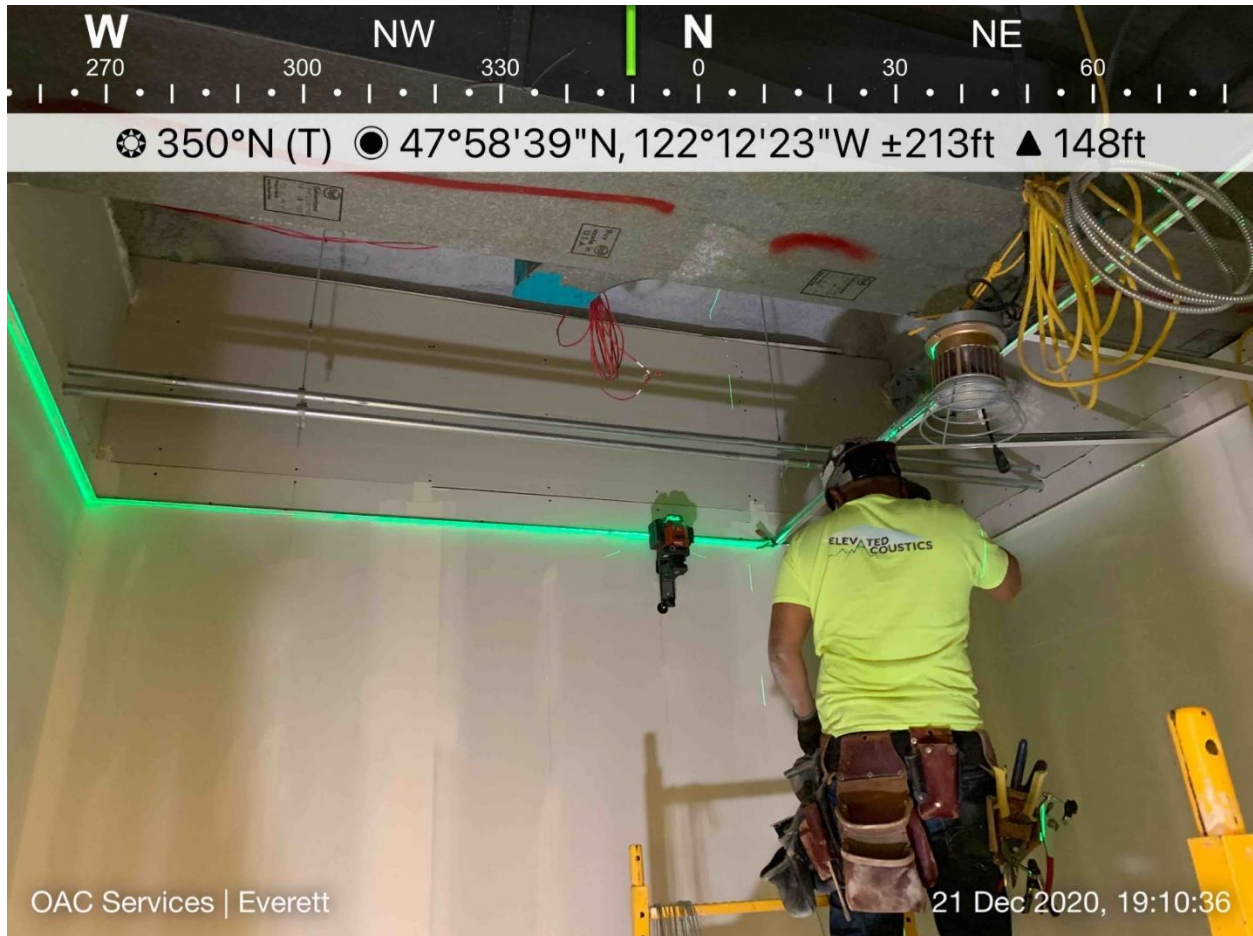
Laying out ceiling grid in a fourth-floor office.
