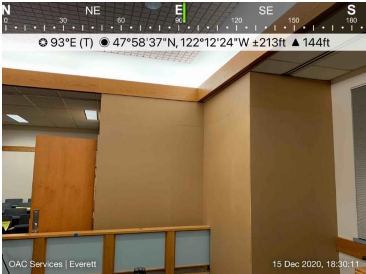
Level 5 shearwall work enclosure.
