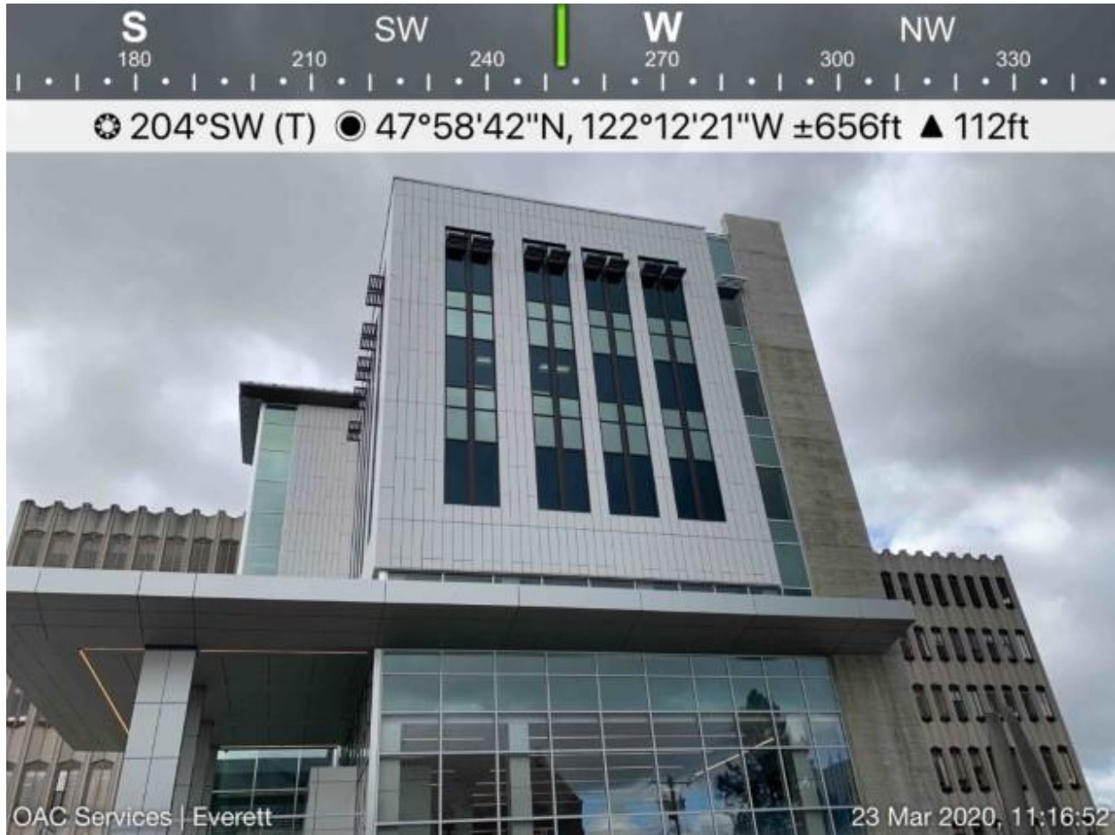
The Snohomish County Courthouse's North Elevation.
