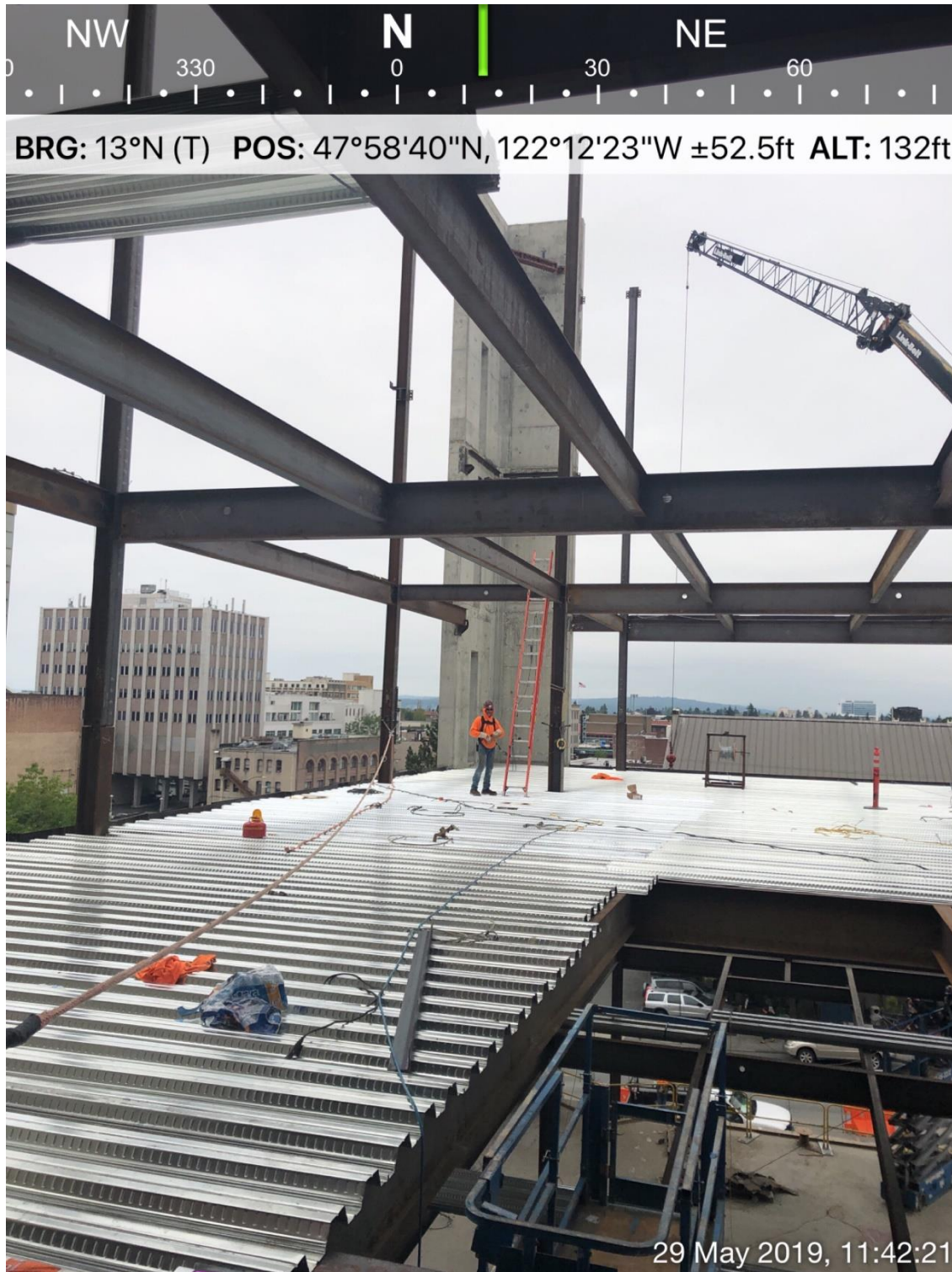
Figure 1: Metal pan decking installation at Addition Level 3, structural steel at Level 4.
