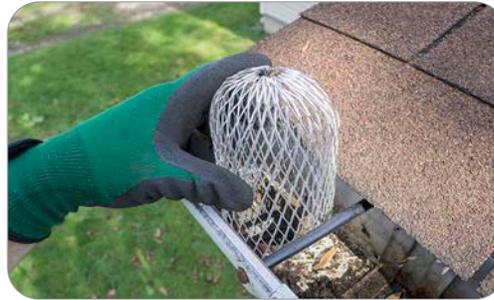
A simple wire mesh or plastic strainer sits inside the downspout inlet and is easy to clean when it fills with debris.
