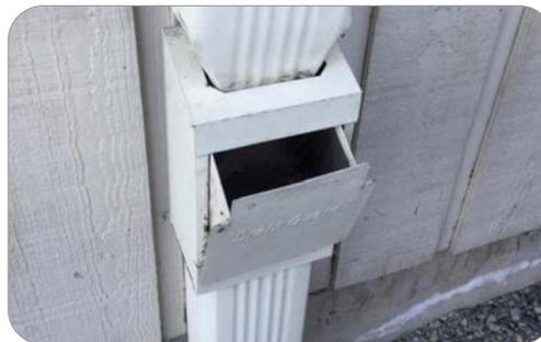
You can retrofit a strainer cup that pulls out of the downspout for regular cleaning and inspection.
