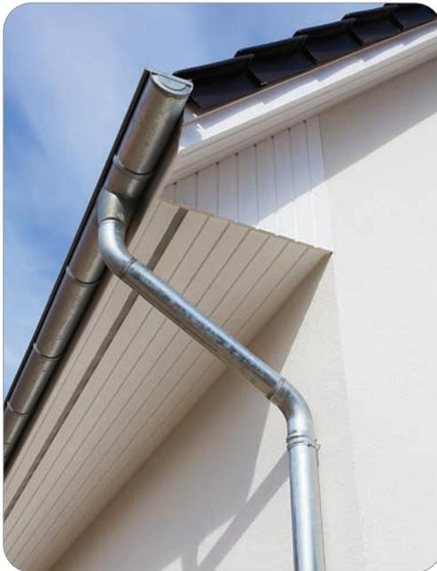
Gutters collect the rainwater that drains from a roof and directs the runoff to the ground via a downspout.
