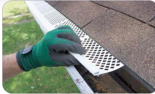
This type of screen covers the gutter opening with a mesh or lid that keeps debris out while allowing runoff water to flow through it.
