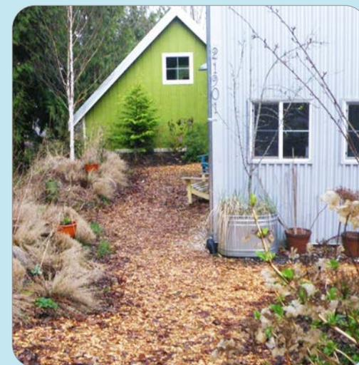
Added wood chip mulch at this roof's drip-line helps prevent erosion and allows runoff to infiltrate.
