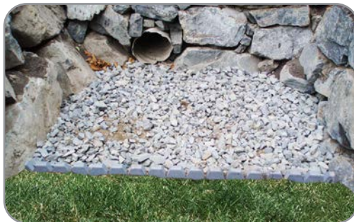
A level spreader is typically a notched board that SPREADS the flow of water coming out of a pipe across a wider area. Often rock pads are placed between the pipe outlet and the spreader board to SLOW the flow.
