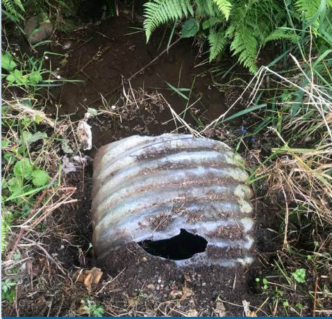
Existing Drainage Pipe
