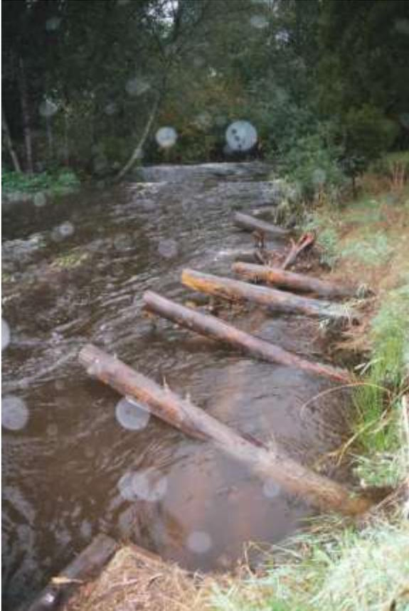
Figure 2. LWD pieces impaled into streambank as part of larger LWD debris jam (27 pieces).
